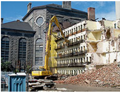
Material recovery in action (Photo: Costello Dismantling)
