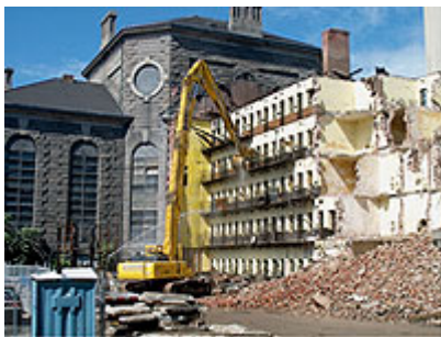
Material recovery in action (Photo: Costello Dismantling)
